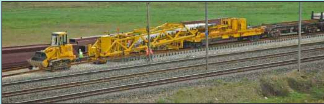
Automatic Track laying machine
