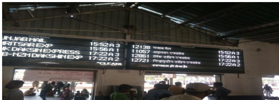
5- line Train Timing Display boards provided at BHS station
