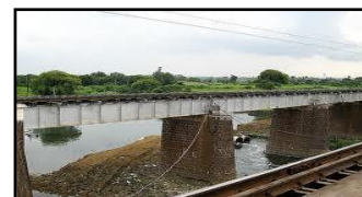
Bridge near Habibganj
