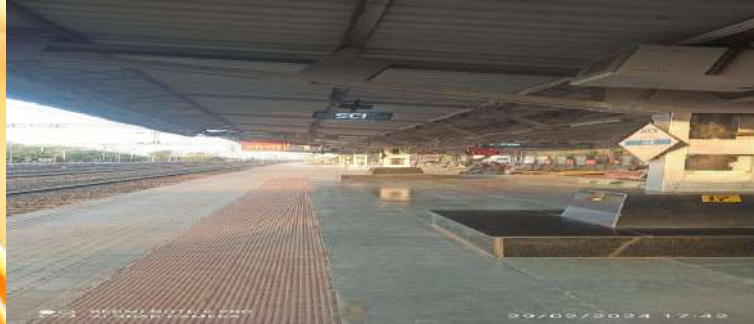
Coach Guidance System at Sachi station
