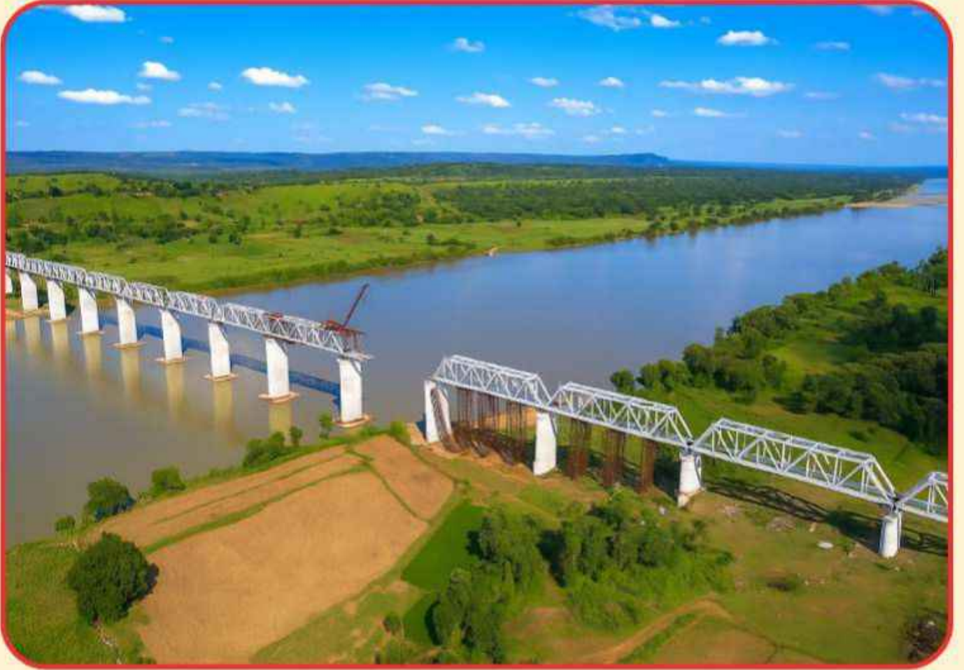
SONE BRIDGE IN REWA-SIDHI SECTION
